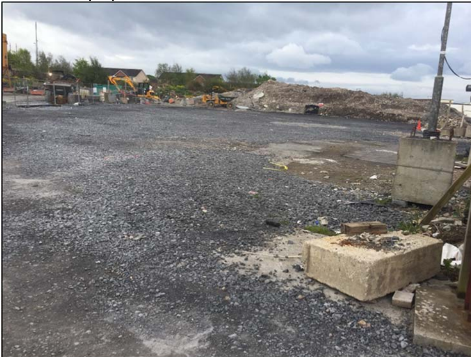
Plate 5-3: Spoil and Bare Ground (ED2)
